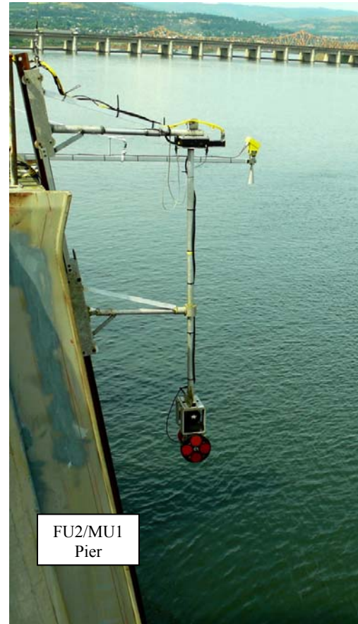
Figure 2.8. Photograph of the ADCP/DIDSON at The Dalles Dam, 2007
